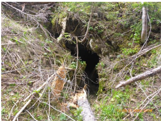
Collapsed shaft (pinge) und portal of the 45 m extending Wohlgemut-gallery northeast of Plonlacke.
