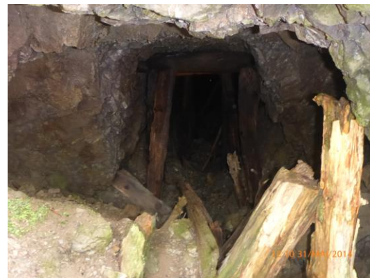
Collapsed shaft (pinge) und portal of the 45 m extending Wohlgemut-gallery northeast of Plonlacke.
